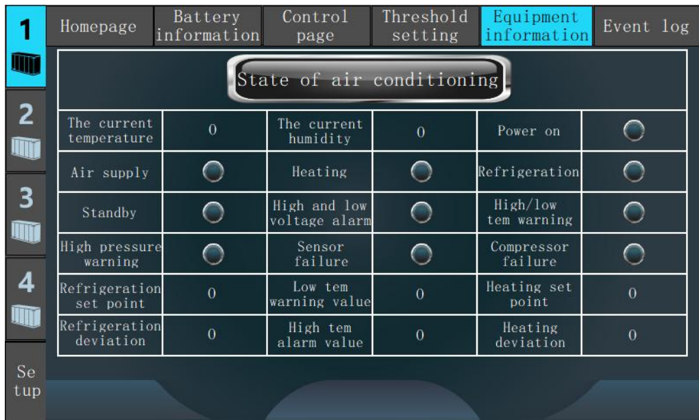
Figure 6-19 Air conditioner status
